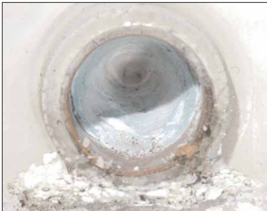
Completely plugged tube.
