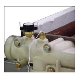
5. Remove the 8 bolts holding the main inlet/outlet head.
